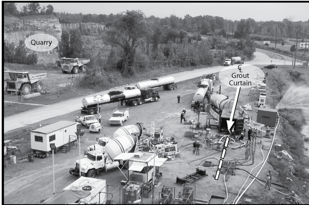
FIG. 6: Project site on Grouting Day
